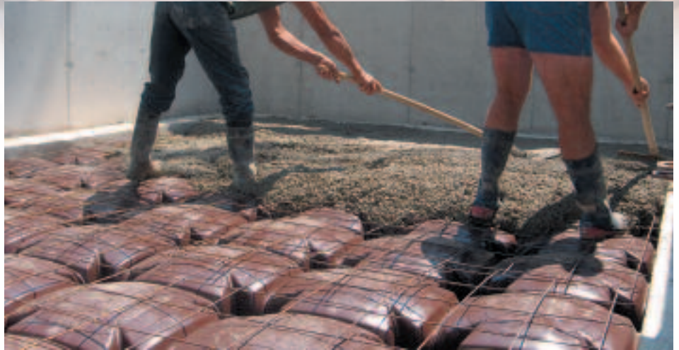
Photo 4 - Casting of the floor
