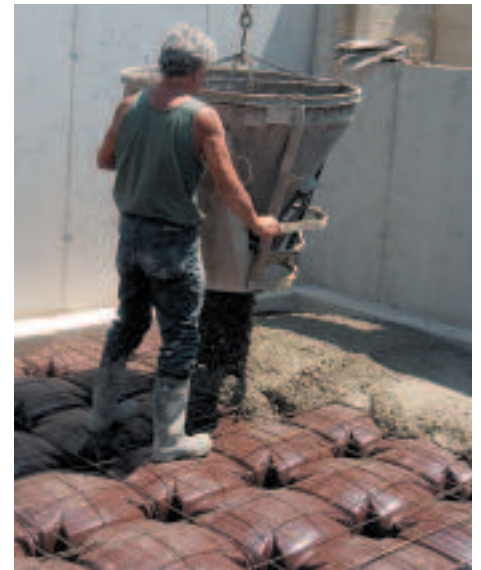
Photo 3 - Casting of the floor
