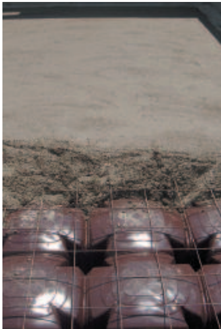
Photo 5 - Casting of the floor
