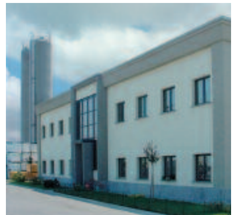
Plant in Stradella (PV)
