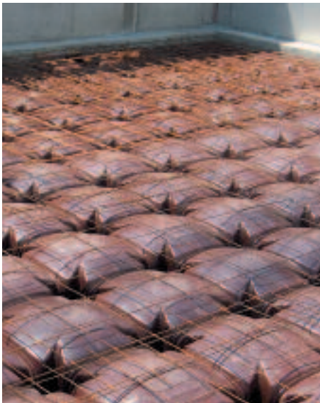
Photo 2 - Laying of Guttadrytek®
